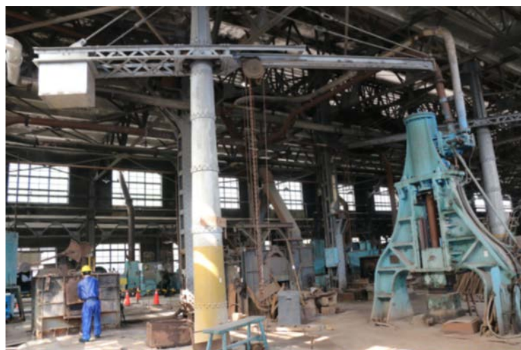
Figure 20. Current conditions of steam hammers (A45) and cranes (A47).
