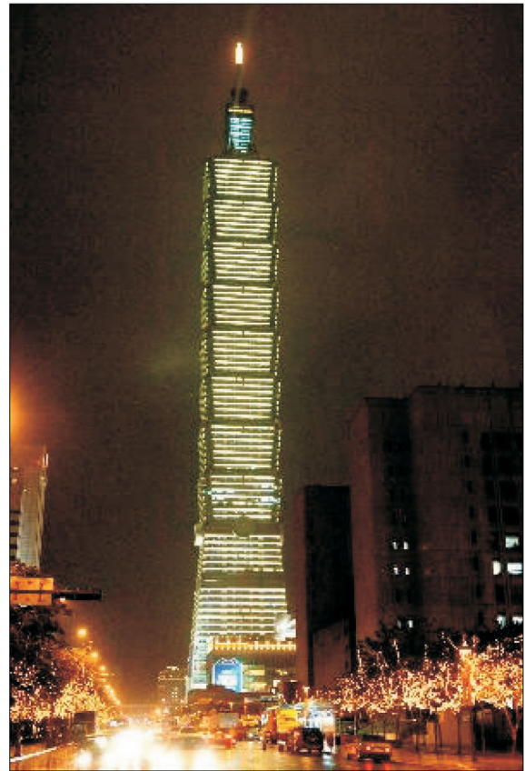
Figure 3. Photo of Taipei 101 Tower.
