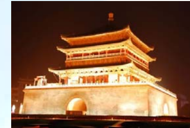
The Bell Tower and the Drum Tower
