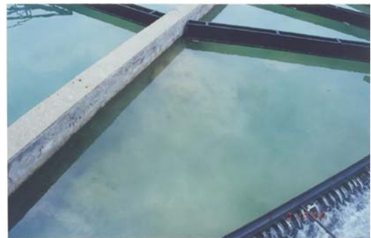
Figure 1. Overturns of the blanket.
